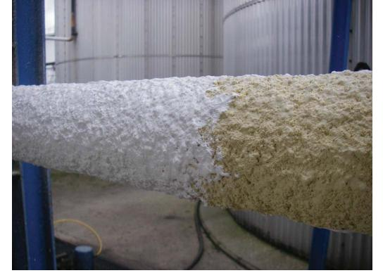
Top coated with **SUPERTHERM** ® for weathering.
