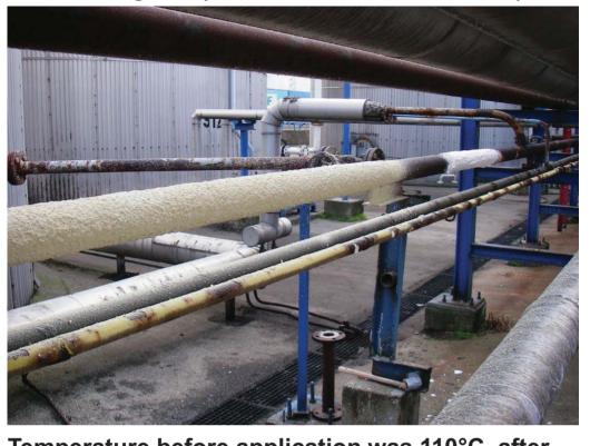
Temperature before application was 110°C, after 6 mm / 236 mils DFT of HPC temperature was 47°C.
