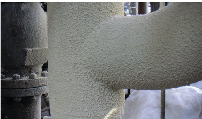
Finished multi-shared HPC® Coating application.
