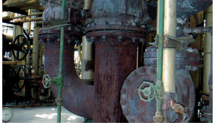
Pipe system before HPC® Coating, extensive CUI.
