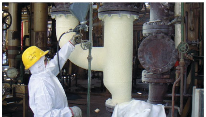
Phase of HPC® Coating application.
