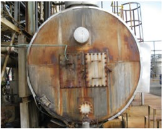
Incinerator before HPC® Coating application was 180°C (356°F).
