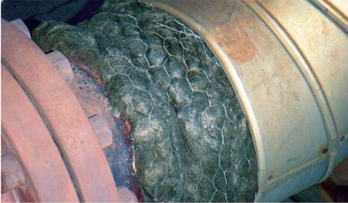
Exposed antiquated insulation.
