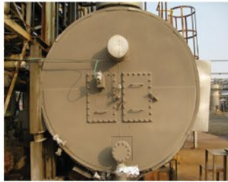
Incinerator after HPC® Coating application was 50°C (122°F).
