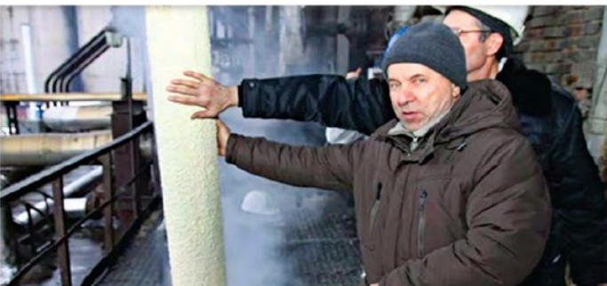
This pipe surface was 467°C (872°F) before coating. These men were able to touch the pipe after only 25mm (1") of HPC® Coating was applied.
