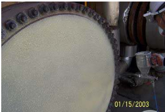
HOT PIPE COATING 1 st Application
