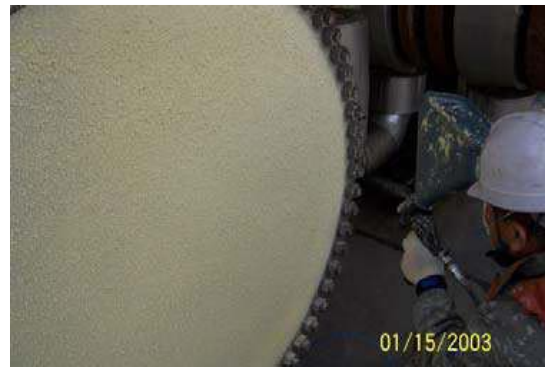
HOT PIPE COATING 2 nd Application
