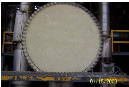
HOT PIPE COATING 3 rd Application (12~15mm thick)
