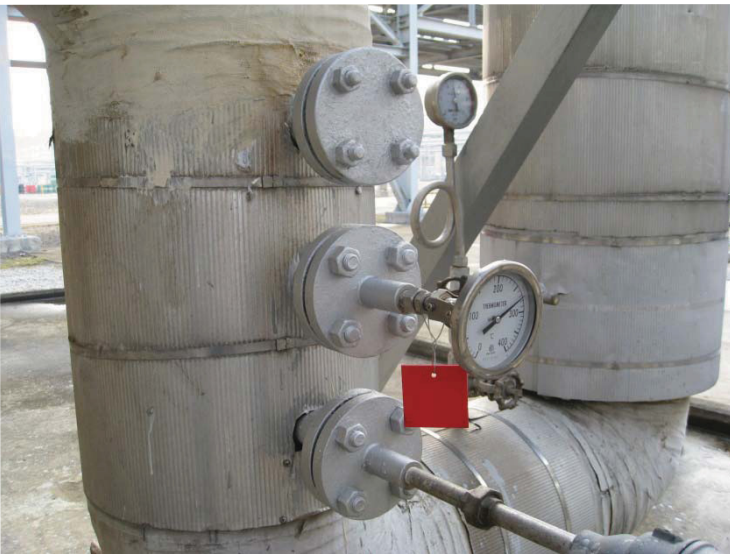
Flange Before coating: 130^{\circ}\text{C}
