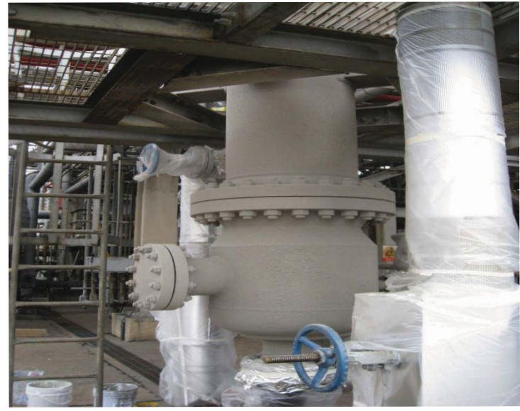
Strainer After coating: 45^{\circ}\text{C}
