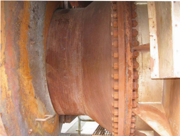
Incinerator Before: 260^{\circ}\text{C}
