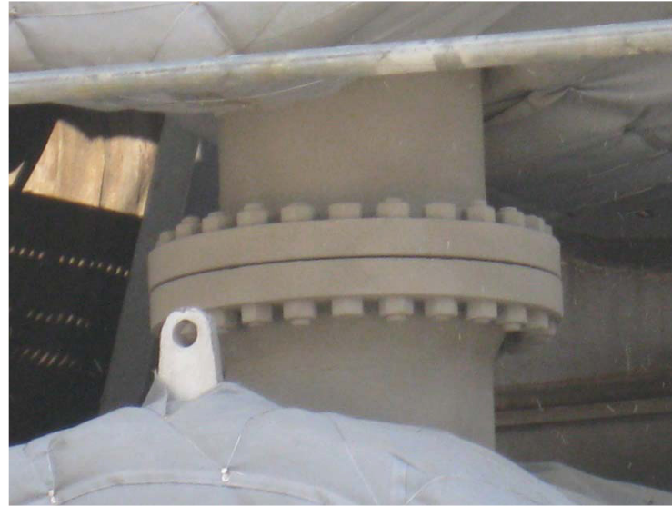
Flange After coating: 55^{\circ}\text{C}
