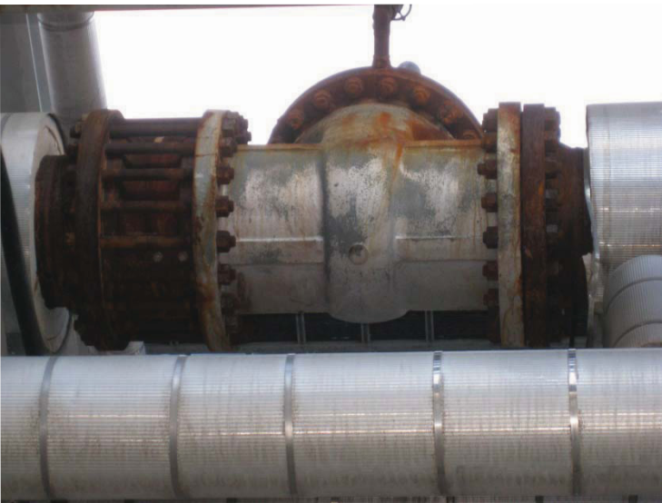
Valve Before coating: 160^{\circ}\text{C}
