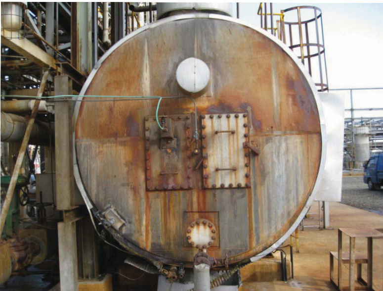
Incinerator Before: 180^{\circ}\text{C}
