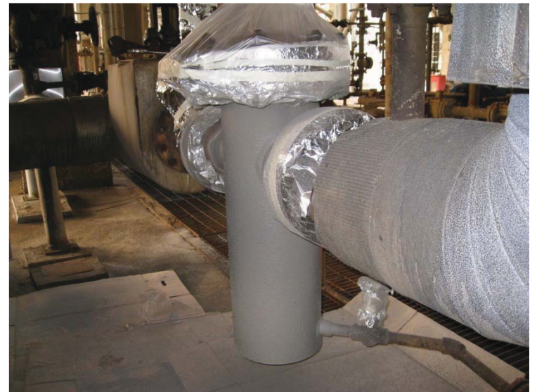
Strainer After coating: 50^{\circ}\text{C}
