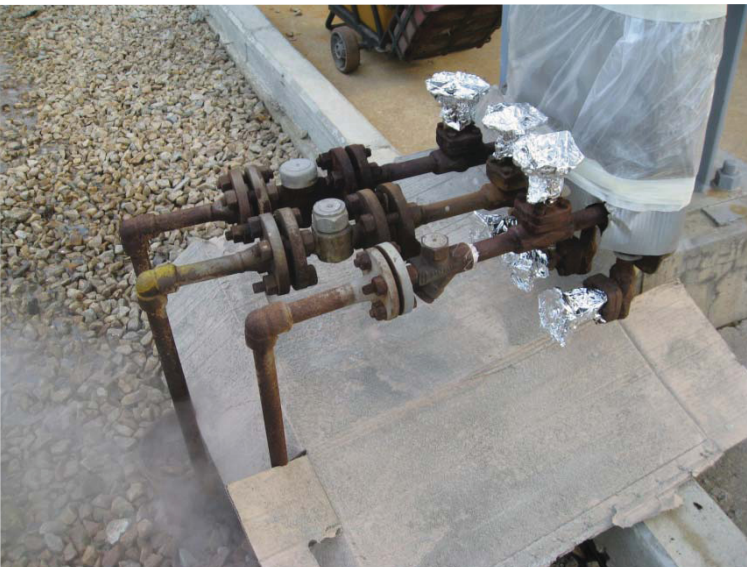
Trap Before coating: 180^{\circ}\text{C}
