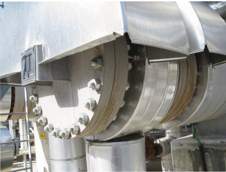
Flange Before coating: 130^{\circ}\text{C}
