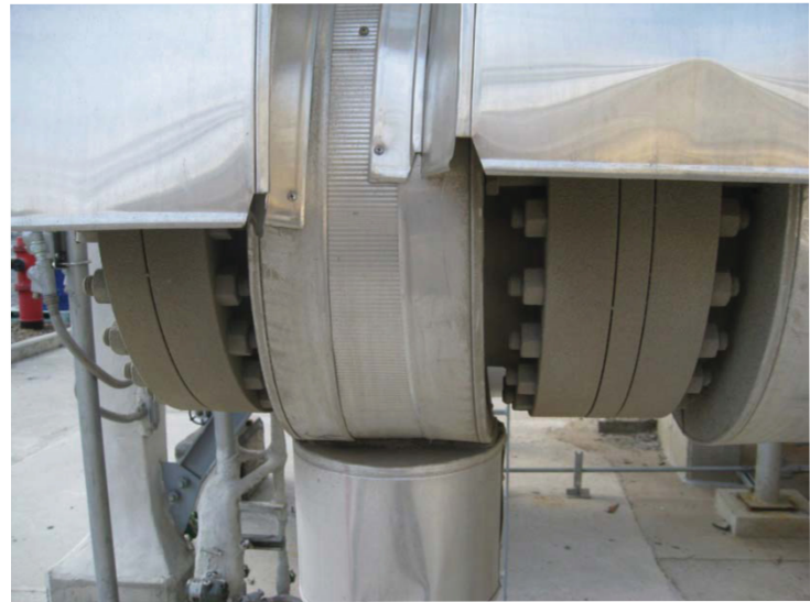
Flange After coating: 45^{\circ}\text{C}
