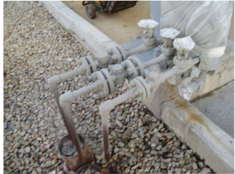
Trap After coating: 50^{\circ}\text{C}
