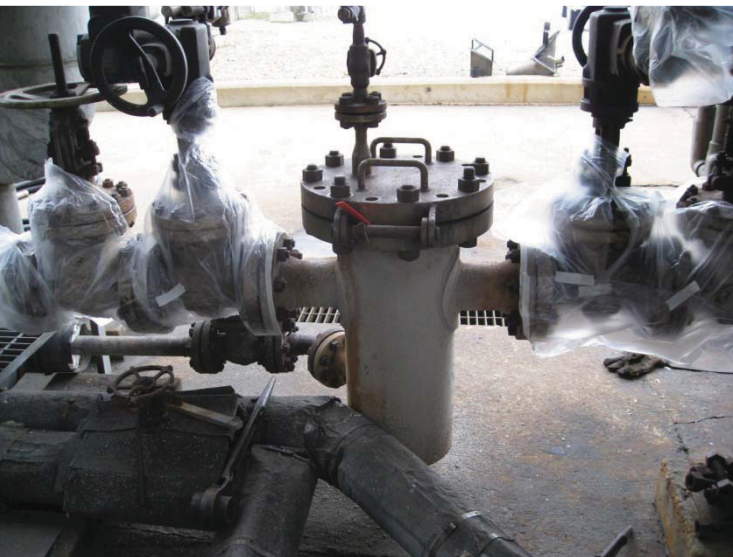
Strainer Before coating: 180^{\circ}\text{C}
