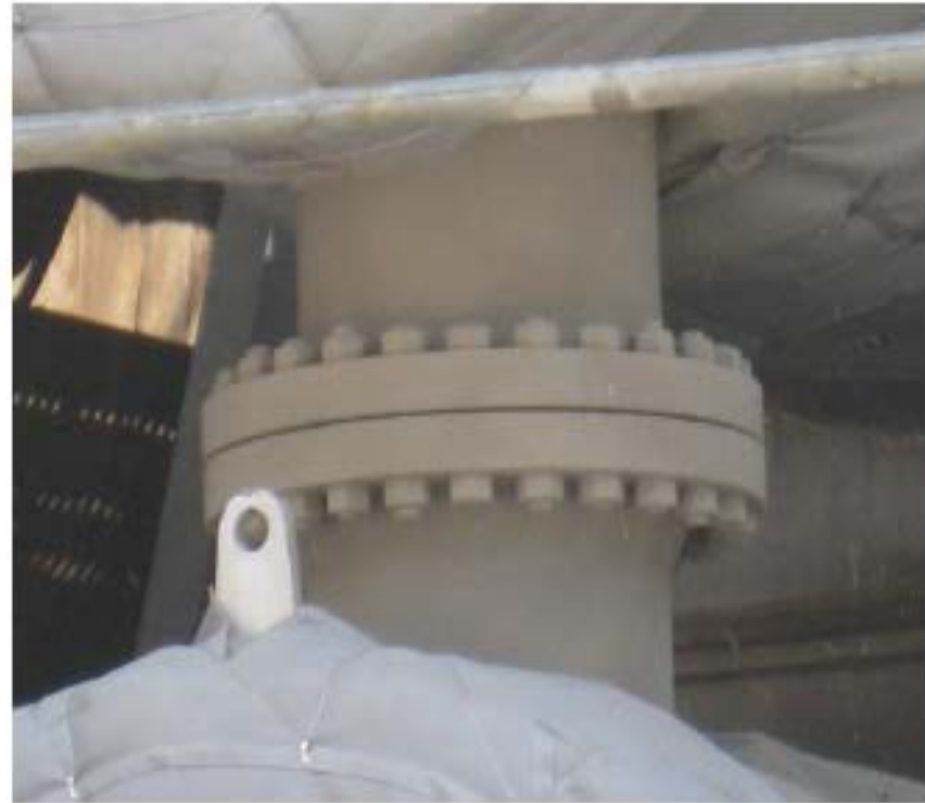
Flange After coating: 55°C
