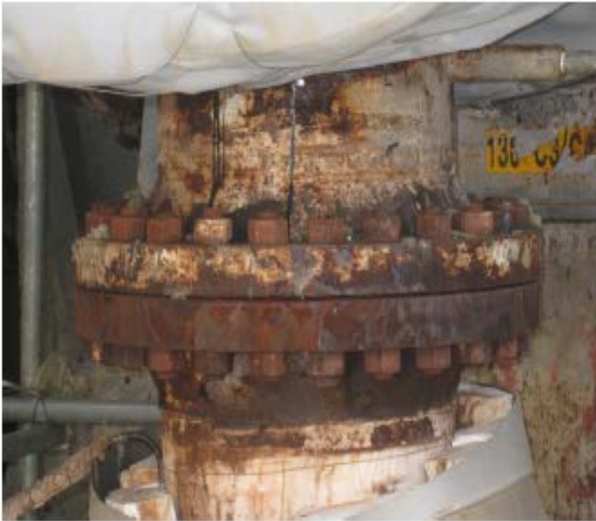
Flange Before coating: 185°C
