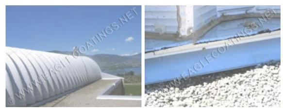
SUPERBASE (HS) ® applied on all bolts and seams at 30SqFt p/gal. The bottom base flashing was applied liberally with added material to accommodate the anticipated ponding water.
