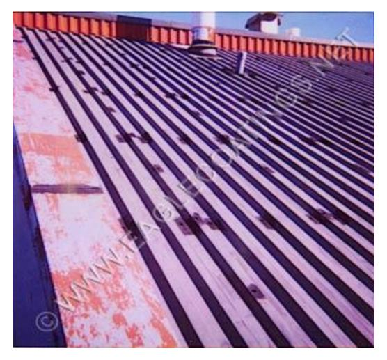
**Solution:** A Function Coating System consisting of <u>RUST GRIP®</u> **Rust and Biohazard Encapsulation** primer coat to permanently seal in the rusting metal
