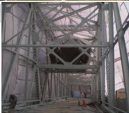
Photos courtesy of Saffo Contractors
