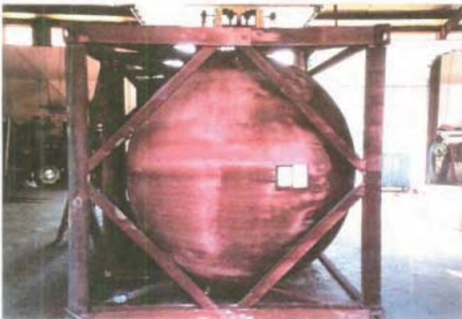
RUSTY TANK BEFORE RUST GRIP APPLICATION
