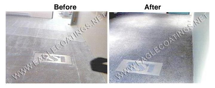
Long lasting High Gloss slip protection that is resistant to water, stains, chalking, solvents, salt etc. Water Based Epoxy was chosen for the lobby because it is not subjected to UV rays and solvent odours were not acceptable.
