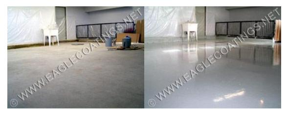
24 hours later **NON-SKID** <sup>®</sup> - HIGH GLOSS, coloured light gray to the owner's specification, was applied in 2 coats cross hatched at a net spread rate of 100 sf per gallon for an outstanding, chemical resistant and low maintenance finish.
