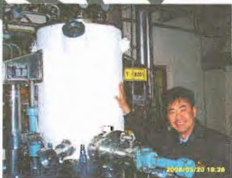
<Checking insulation effect again>
