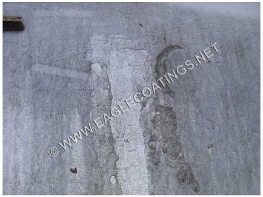
An additional 8 mils WFT = 5 mils DFT of <u>SUPERTHERM</u> ® was added over the whole roof.
